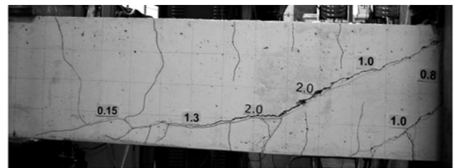
(a) Vertical cracks due to negative moments, SS1b-1
