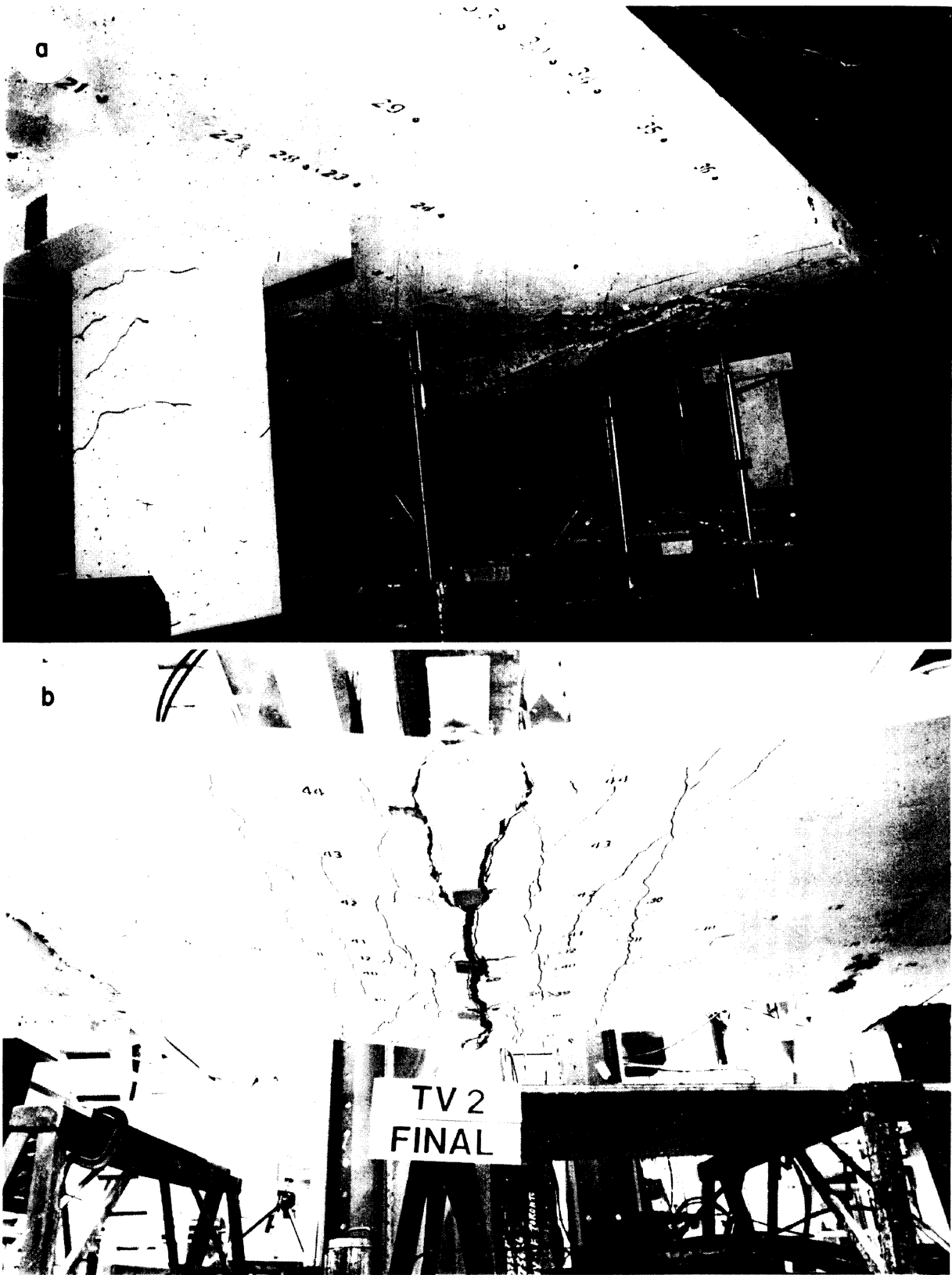
FIG. 6. Slab specimens after failure: (a) punching failure of slab TV1; (b) failure of slab TV2 due to rebar rupturing.
